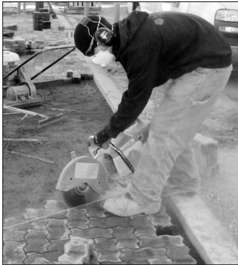
Jonathan Gallant, a labourer with Red Oak Landscaping, cuts the bricks for the inter-locking sidewalk on Queen Street in Charlottetown. (Smith photo)
